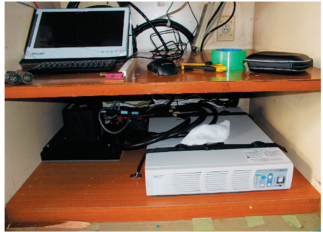
Photo 4. IMU (lower left) and UPS (lower right) installed on the lower part of the observation equipment rack of S/V Uzushio .
