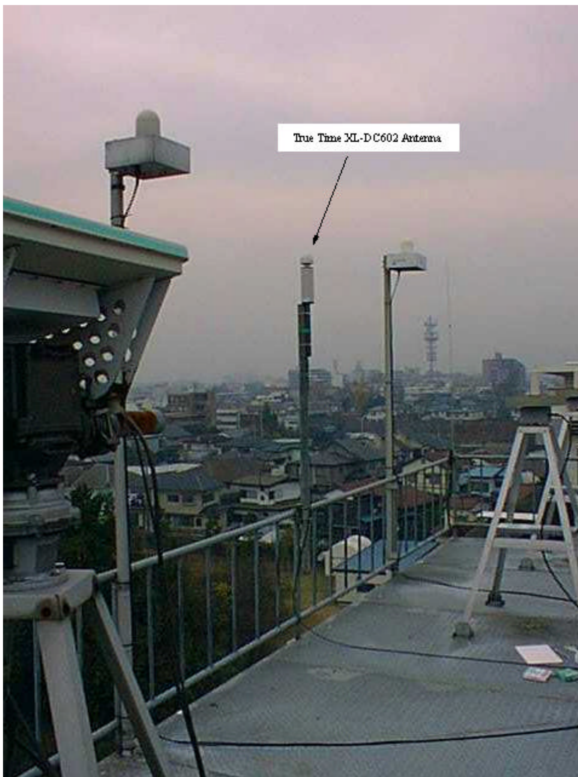
Photo 1. Antenna setting at the Communication Research Laboratory rooftop.
