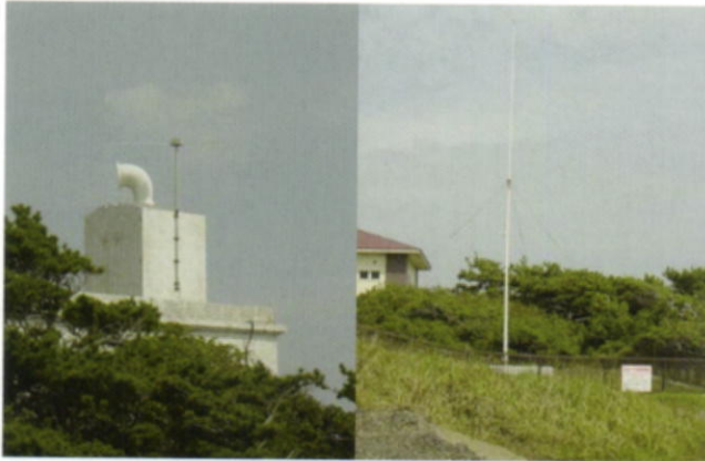
Nojima Saki Ocean HF radar station (Left: receiving antenna, right: transmitting antenna)
