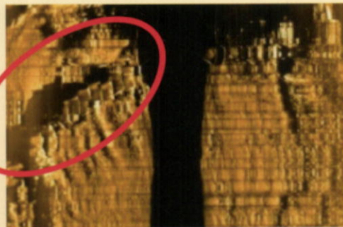
The damaged breakwater at Port of Ofunato
