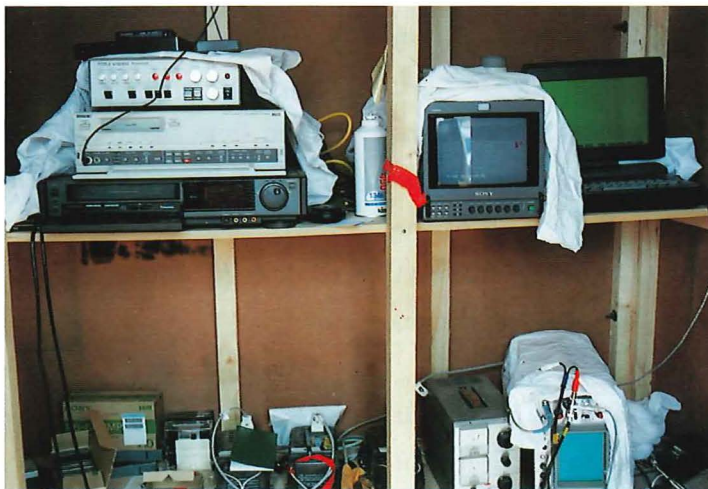
Photo 3. The recording equipments.
