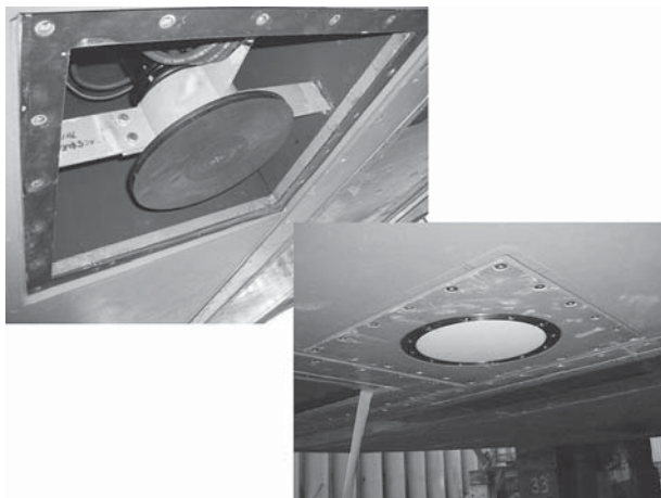
Photo. 2 Installation of the acoustic transducer under hull of the S/V "Takuyo".
