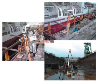
Photo 5 Measurement of the distance between the acoustic transducer on the bottom of the vessel and the GPS antenna at the mast.
